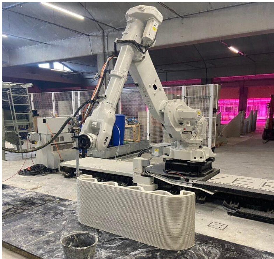
Figure 3 A large-scale concrete 3D printer at work. The concrete is extruded in layers by a robotic arm. This method can build walls and structures on-site rapidly. (Source: Wikimedia Commons.)
